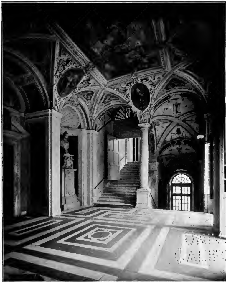
STAIRCASE IN THE PARODI PALACE, GENOA.
